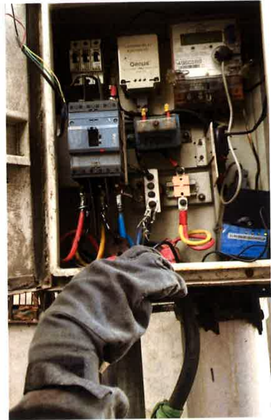
Hooking removal from Meter Pillar Box
